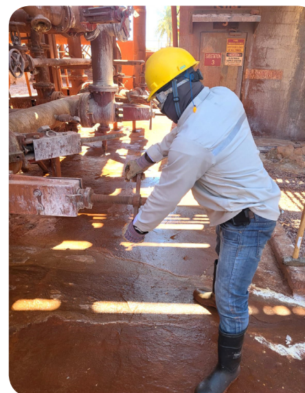
Hopeton at work closing a discharge valve.
