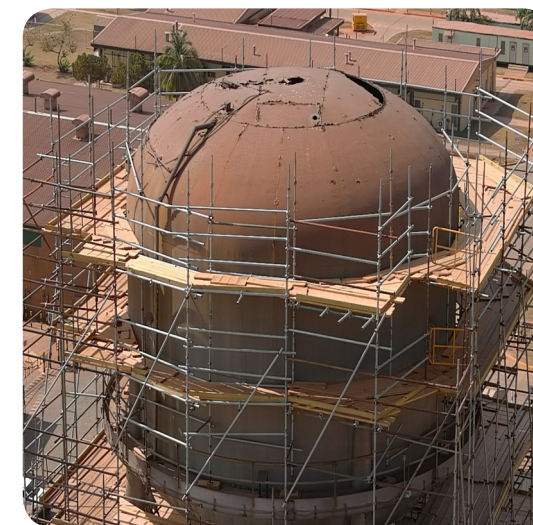
The general water tank undergoing repairs.
